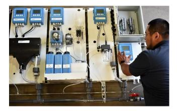
From intake through flocculation, sedimentation, filtration, and disinfection, water plants monitor and control a number of water quality parameters before going to distribution. Increasingly plant managers are recognizing the value of a final check on those parameters. A mid-size water system in the southeast was looking to pull together multiple measurements in a single panel. After reviewing off-the-shelf solutions, they realized there was nothing that met their requirements.
