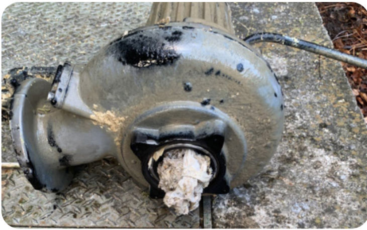
Depicted above is a clogged submersible pump typical of the issue experienced in the original prison submersible pumping station confined space wet well. The operations staff was faced with removing the pump for clog removal every two days. Unfortunately it had become an expensive and time consuming nuisance.
