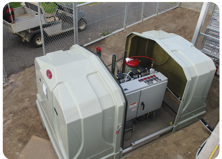
The EVERLAST™ above-ground pumping station at the prison simplifies operator access and eliminates confined space concerns by mounting a complete lift station at grade level in a quick-access enclosure. All pumping and control equipment is safely accessible by a single operator, significantly lowering O&M time, hassle and cost.
