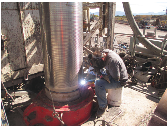
Welding the well screen
