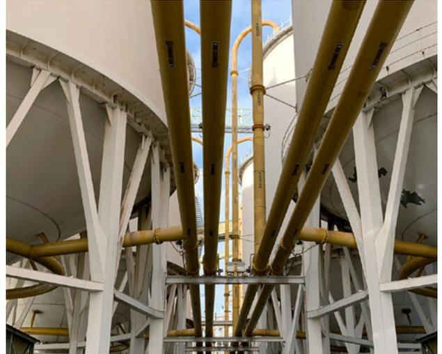
*Figure 1: Silos with fumigant piping*
