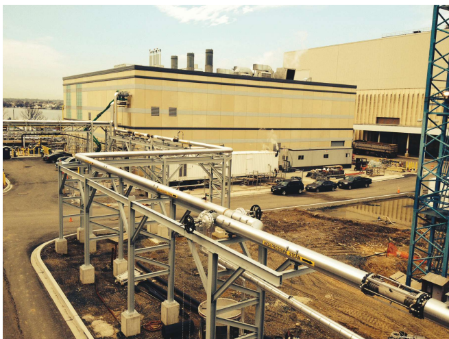
New CHP facilities at the Blue Plains Advanced Wastewater Treatment Plant in Washington, D.C. enable DC Water to maximize energy recovery while also producing steam needed to drive THP.
