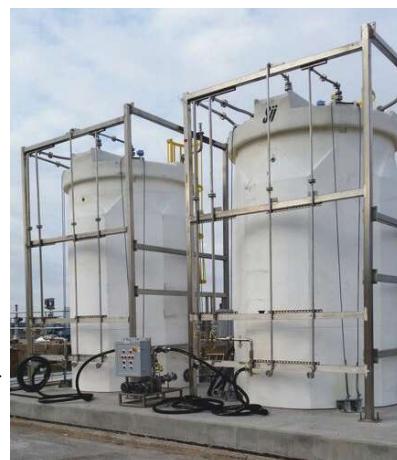
Figure 3. Temporary bulk PAA tank installation used for full-scale pilot testing at the Stiles WWTP in Memphis, TN. (Credit: PeroxyChem)
