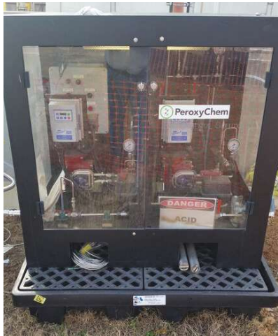
Figure 4. Typical pump skid used for PAA feed. (Credit: PeroxyChem)
