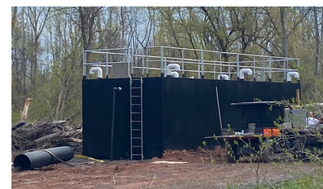
A modular treatment plant shipped to site and specified to meet permit limits. Plumbing is attached and electrical service provided to begin treating effluent.
