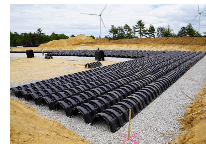
Large subsurface dispersal systems are practical solutions for communities. These systems provide additional benefits of polishing and aquifer recharge.
