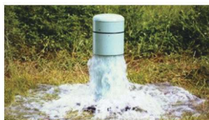
HG-1 Flushing Unit Installed
