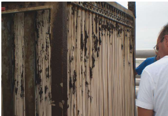
A cassette is lifted from the MBR process to clean off solids.
