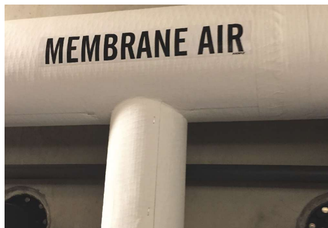
Air is introduced for scouring the membrane surface.
