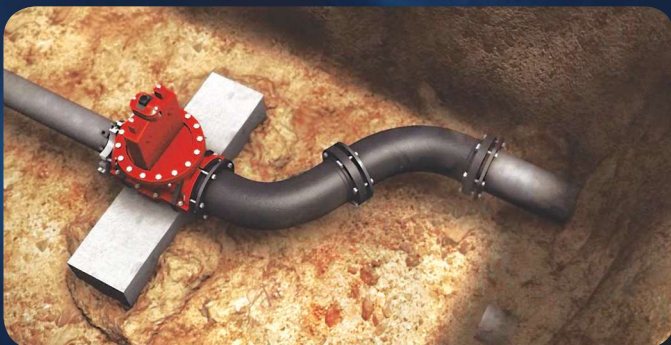
New, larger diameter pipe connected
