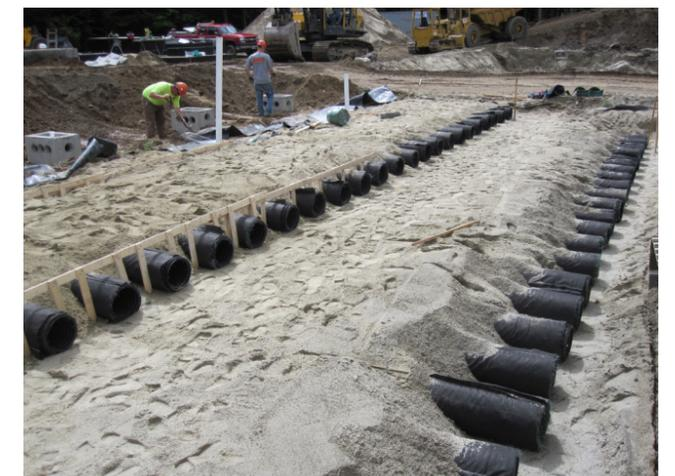
Pipe bundles in the double-stacked configuration are properly spaced.
