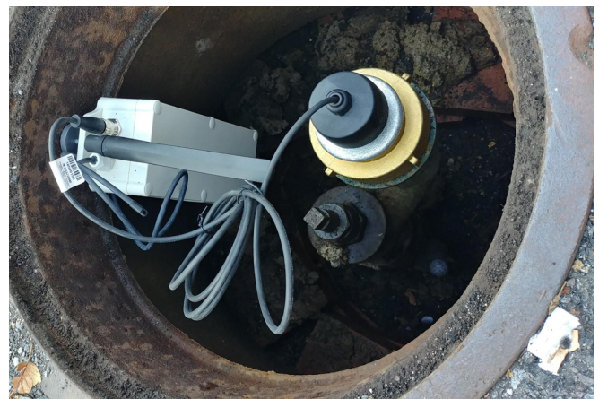
Figure 2. AQS underground acoustic sensor installation
