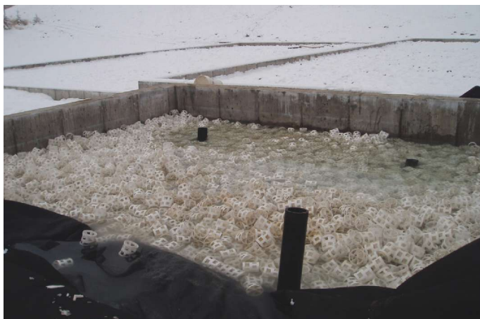
Figure 3. Attached-growth media system
