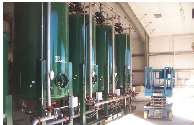
Figure 2. Treatment with ion exchange resins
