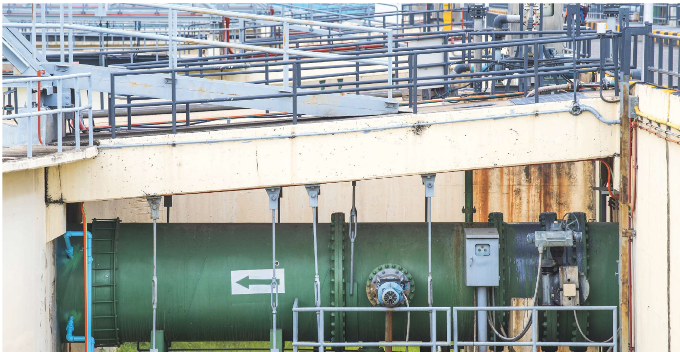
Input raw water pipeline travels to the solid contact clarifier tank.
