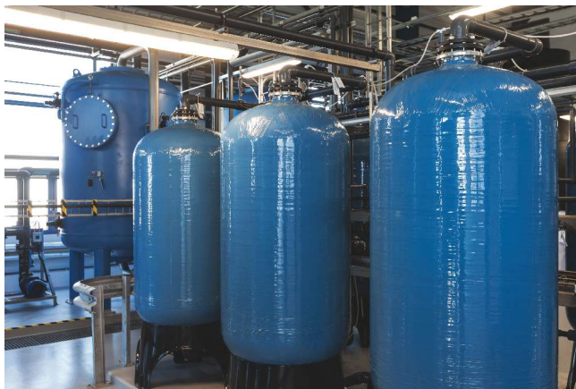
Filtration tanks for biological activated carbon treatment.
