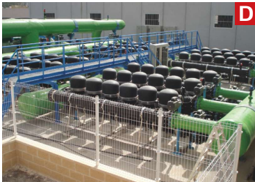
Spain SWRO Desalination Plant, UF Pre-filtration
