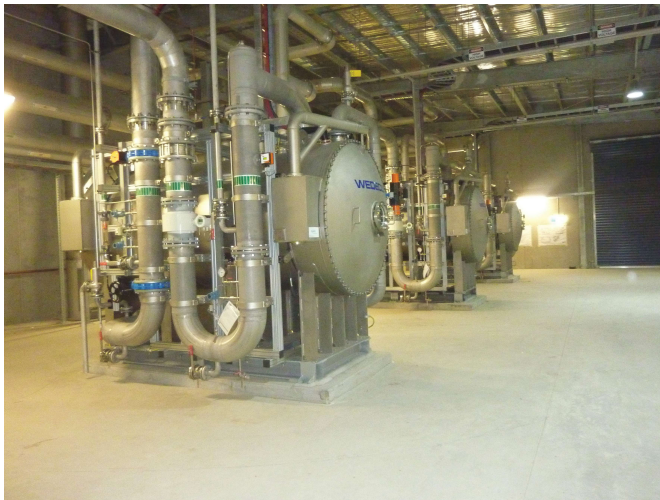
Figure 3. Melbourne Water uses these ozone generators as components for treating secondary effluent at its Eastern Treatment Plant at Carrum, using a pre-ozone/biological media filtration/postozone/UV/chlorine process train to improve discharge quality and produce water suitable for horticultural irrigation and potential third (purple) pipe domestic use.
