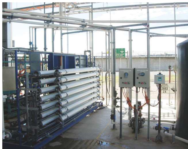
Figure 4. A pilot plant was built at Luggage Point, Brisbane, to check the MF/RO technology before the full scale Advanced Water Treatment Plants were built, highlighting the need to recognize that influents to recycling and desalination plants can vary considerably.
