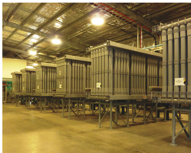
Figure 2. The Glenelg Wastewater Treatment Plant generates recycled water with these ultrafiltration modules followed by advanced oxidation (UV and chlorination) with the consequent saline stream piped to the much larger Bolivar plant for further treatment.
