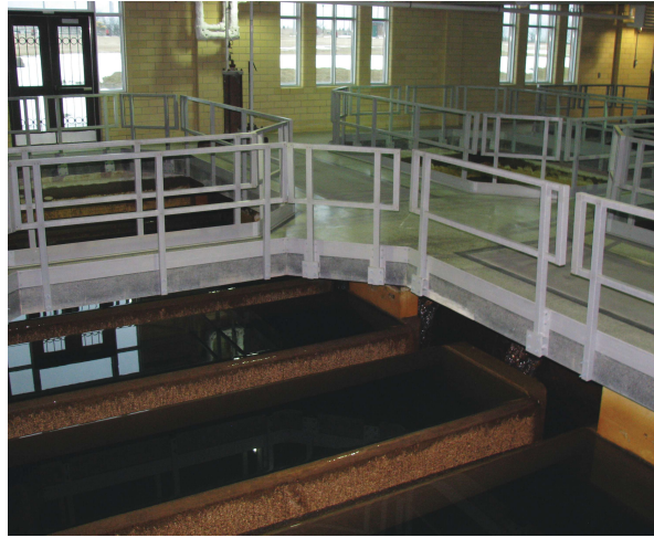
Postfilter disinfection with granular activated carbon (GAC)
