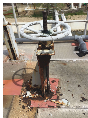
Figure 1. Corroded valve and bar screen at monitoring site headworks
