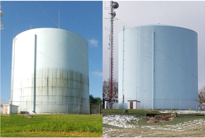
Before and after images showing the thermocline layer eliminated by effective mixing.
