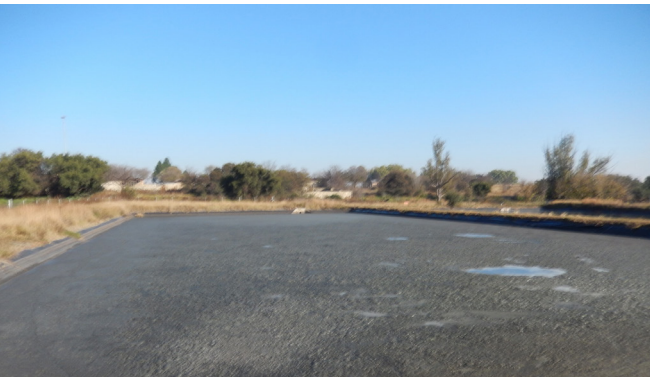
An anaerobic lagoon at a pig farm that has an extensive solid sludge layer on the top.
