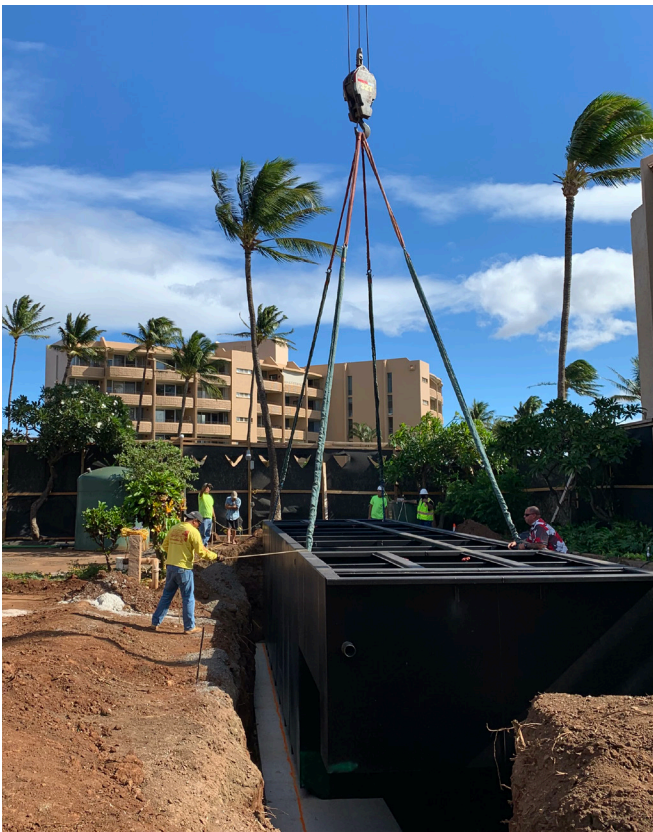
When the Lauloa Maalaea Resort in Hawaii was required to update its wastewater treatment unit due to tighter effluent requirements required in a forthcoming permit update, the new system had to maintain the same footprint of the existing below-grade treatment unit that was being replaced.
