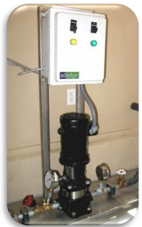
Recycle Pump Skid
