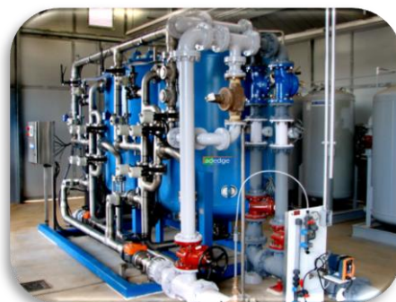
AD26 Iron, Manganese Treatment Skid
