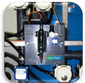
In-line Chlorine Monitor
