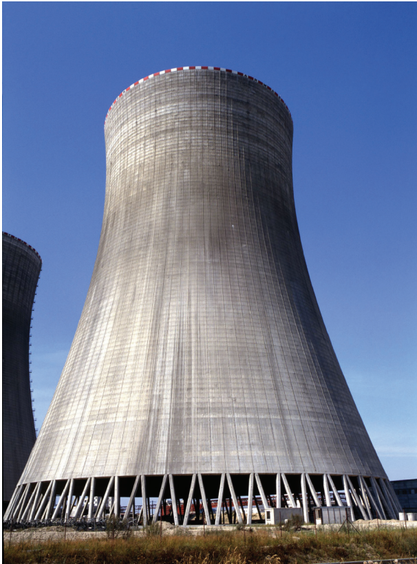
Figure 2: Electric Power Generation Plant Water Cooling Tower
