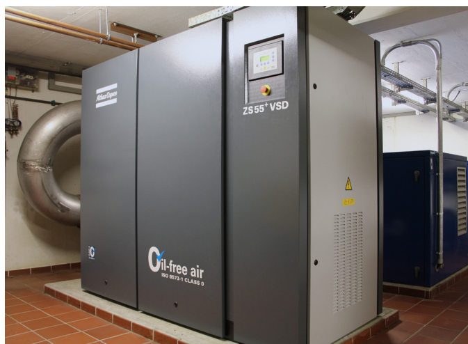
Fig. 2: Compressor station for the seepage water treatment installation. In the foreground, the new speed-controlled screw blower ZS 55+ VSD, which already runs significantly more efficiently than rotary lobe blowers due to their design.
