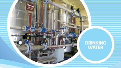
FERAZUR®/MANGAZUR®/NITRAZUR™ is a biological filtration process for the removal of iron, manganese, arsenic, ammonia and nitrates from ground water sources. The precipitate is removed by using Biolite™ "S", our specially developed media that requires no replacement. The bacteria remain in the media even after backwashing, allowing continual operation for indefinite time periods.
