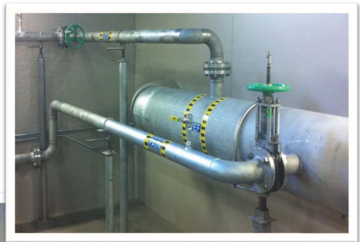
Figure 2: SDOX® Installation Demonstrating Small Footprint and In-Pipe Injection
