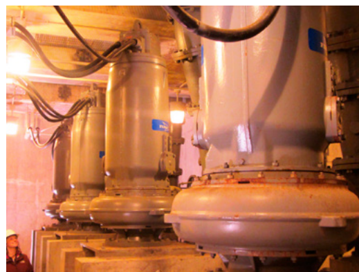
The new N-pumps installed.
