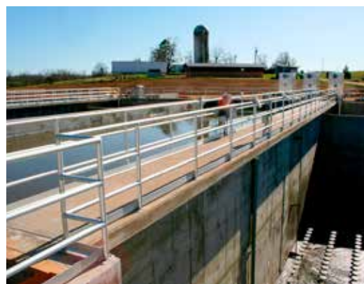
Four new ICEAS basins were constructed for the upgrade.
