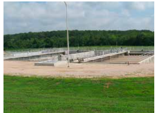
Sanitaire's ICEAS Continuous Flow sequencing batch reactor was selected.
