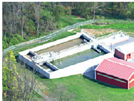
The Newville Borough Water & Sewer Authority SBR tank.
