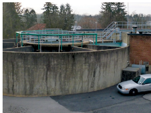
The former package plant system tanks now converted for sludge treatment.
