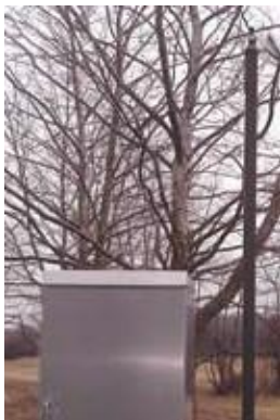
The Telog RTUs used for this project were provided with solar power, eliminating the need for AC power or field visits to change batteries.
