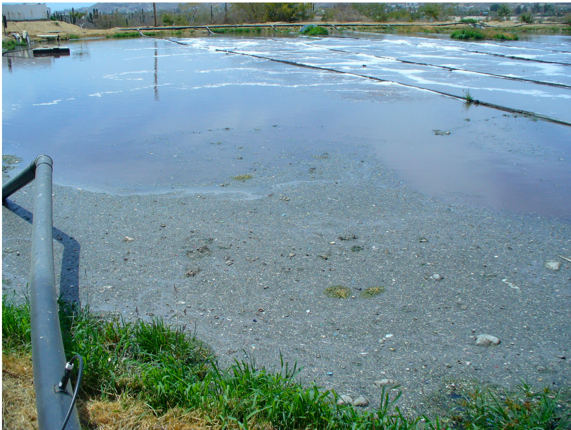
Figure 1 – Short circuited lagoon with exposed sludge buildup around the edges.
