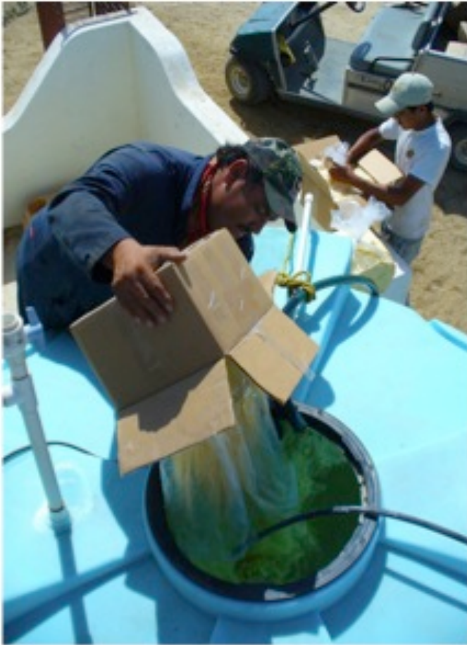
Figure 3 – Premixing of the granular Sewper Rx sludge digestion product was performed in a 25,000 tank prior to pressure injection of the hydrated bacterial solution into the sludge.
