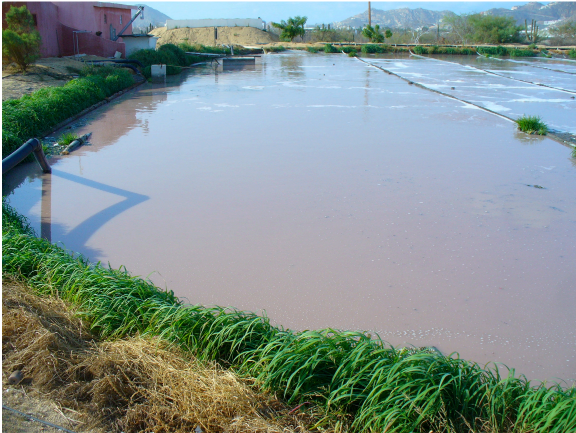
Figure 5 – A photo from the exact same location as Figure 1, taken approximately 70 days following treatment of the raw sludge by the Sewper Rx bio-augmentation blend of bacteria.
