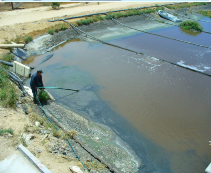
Figure 4 – Pressure injection at many depths into the sludge was performed by technicians. Each lagoon took approximately 7 days for complete inoculation.
