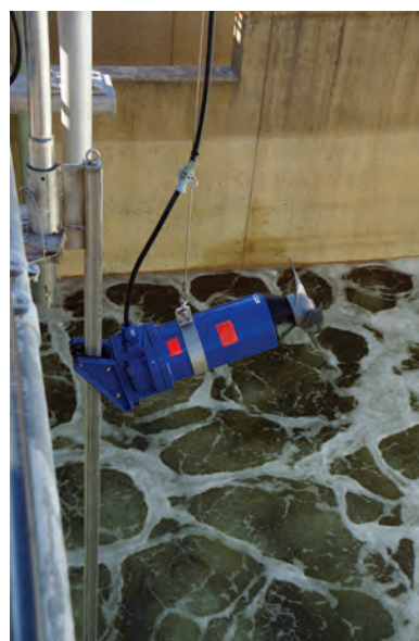
Fig. #12 - Hartford County, MD WWTP utilizes > 100 submersible mixers for various applications
