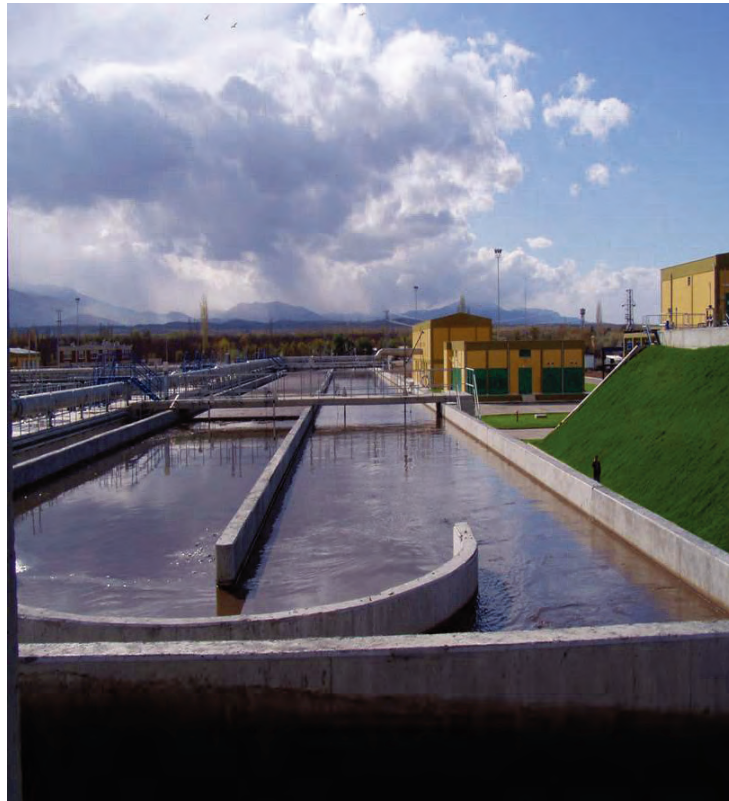
Fig. #19 – Typical Oxidation Ditch (Malatya Turkey)
