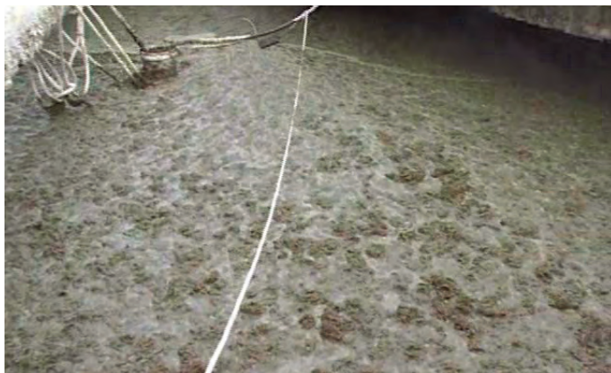
Fig. #11 - Anaerobic Digester Sludge - After Mixing
