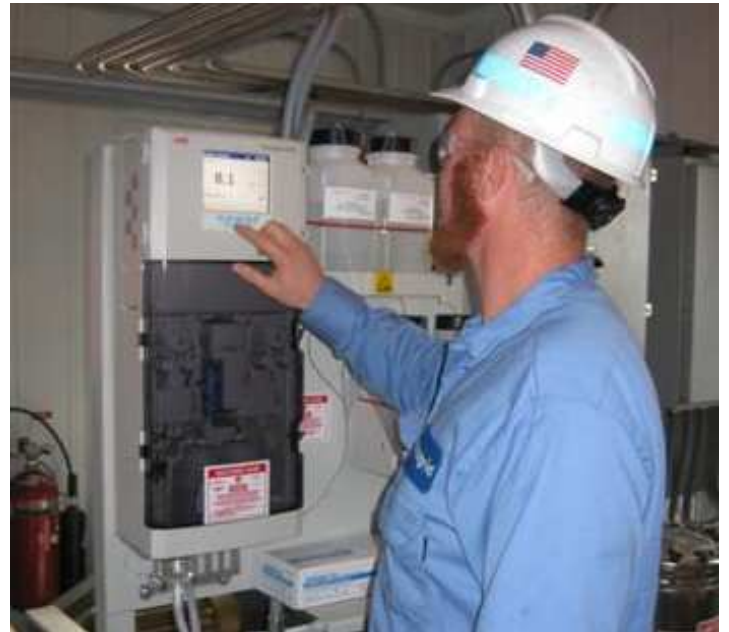
Figure 1. ABB Navigator 600 analyzer monitors silica for new water injection system.
