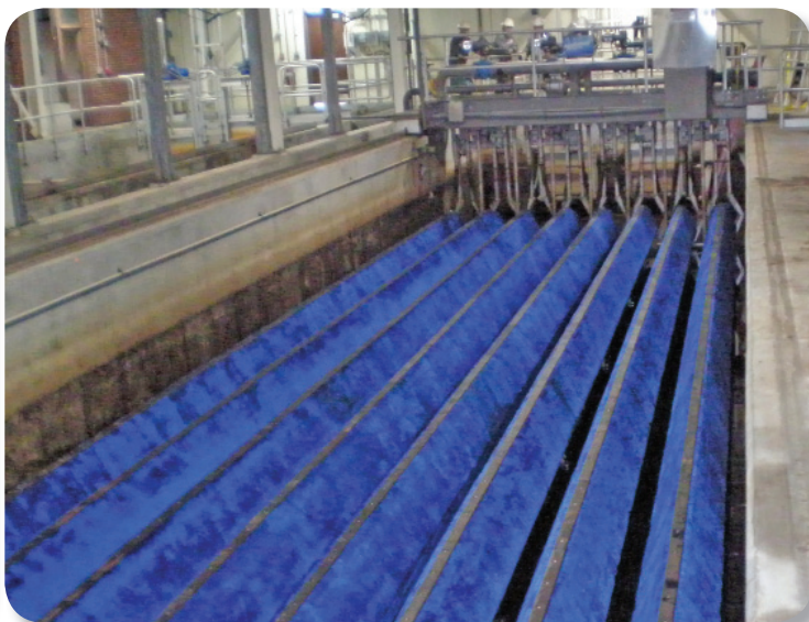
An AquaDiamond® filter with Microfiber cloth polishes phosphorus to < 0.1 mg/l.
