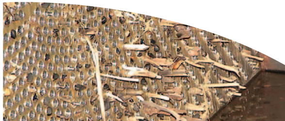
Condenser tubes without debris filter
