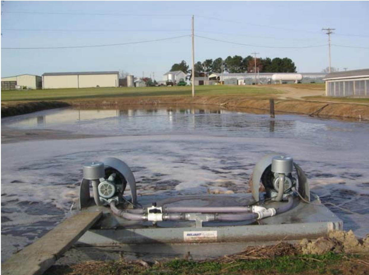
**Figure 2:** Reliant Model WQA Water Moving Aerator located in one end of the hog lagoon. Photo was taken approximately 15 days after aerator startup.
