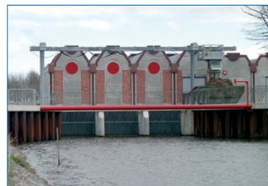
Fig. 2.7-i: Pump station with automatic screens
