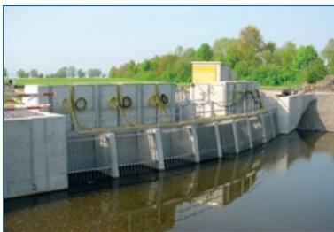
Fig. 2.7-a: Coarse screens upstream of an Amacan pump station (water abstraction from a river)
