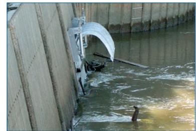
Fig. 2.7-b: Screens with automatic cleaning devices
