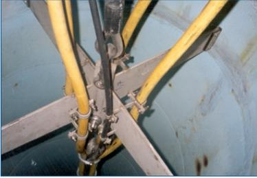
*Fig. 3.3-d: Supports for cable guidance in the discharge tube*
