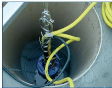
*Fig. 3.3-e: Cable attachment using simple cable straps*
