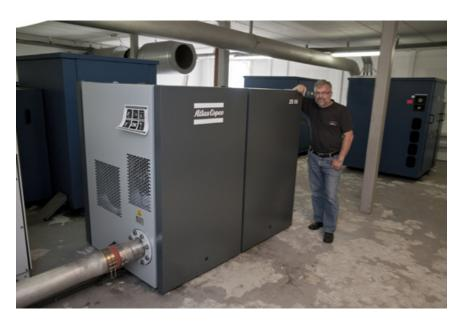
In May 2011 Atlas Copco delivered a new 55 kW variable speed drive blower operating at 0.7 bar(e) to Skanderborg WWTP, replacing a 75 kW lobe blower in one of the aeration process lines.
