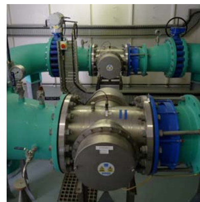
ETS UV model SX installed duty/standby
