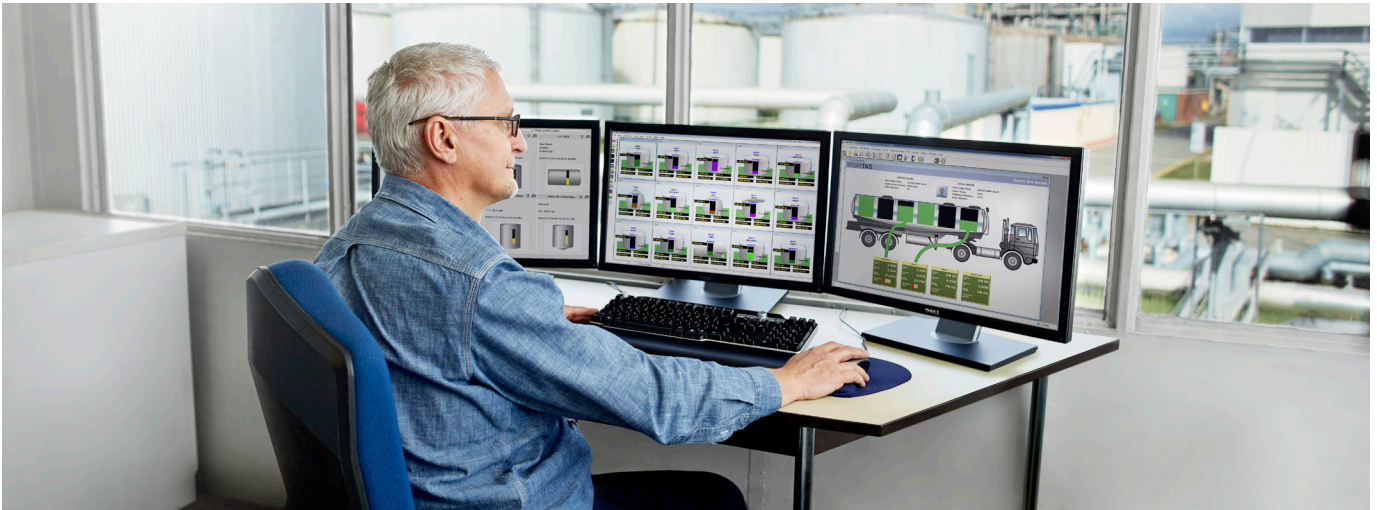
Figure 3: Tank monitoring HMI software, such as Endress+Hauser's Tank Vision, displays the output of each tank in a tank farm and checks for indications of leaks or overfilling.
