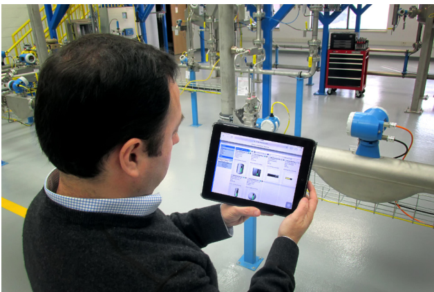
Figure 4: Web server capability lets engineers and operators monitor tanks and receive alarms at a mobile device.
