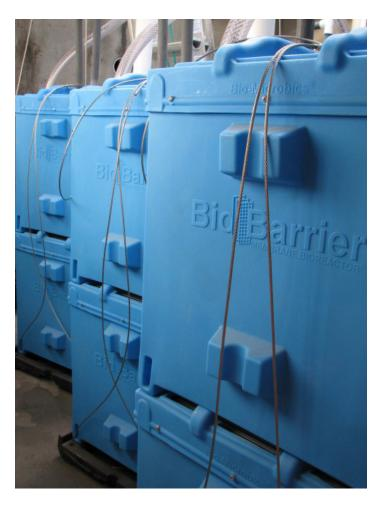
bioreactor acts as a batch reactor and knows when to cycle on and off. The activated sludge provides the bacterial treatment while the membrane provides the physical treatment. Additionally, all electrical systems are tested and certified to <u>U.L., C.S.A, and C.E.</u>
