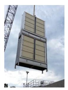
When out of the tank, the construction of the membrane module further enhances the ability to maintain the system in the particular event where circumstances have allowed the spaces between the sheets to fill with sludge which can act to stick adjacent sheets together like glue. In the K-120C and K-240C membrane modules, individual membrane sheets are held together by compression from the
