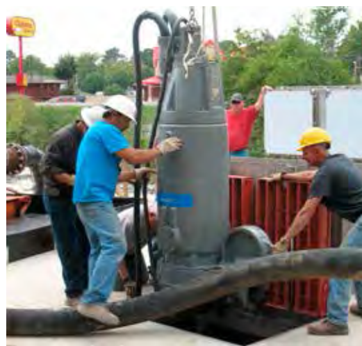
Installation of a Flygt N-Pump at the Fairwood Lift Station.
