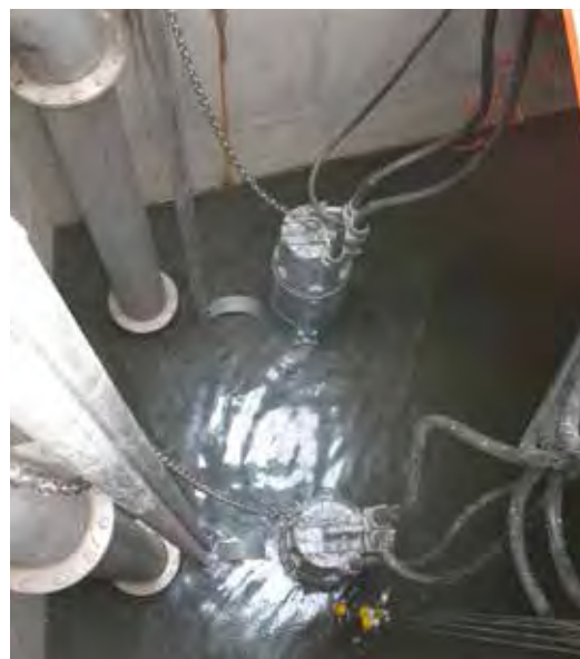
Overhead view of a installed Flygt N-pumps.
