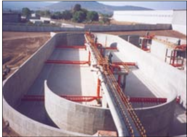
This MTS jet aeration system installed north of Mexico City, Mexico serves a textile plant with a 35-ton-per-day BOD removal requirement.
