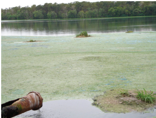
Figure 4 – Numerous sludge islands at the inlet of a 60 acre wastewater lagoon in southern Louisiana.
