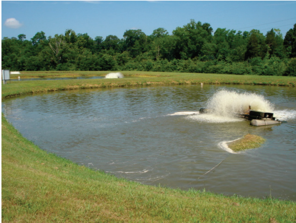
Figure 2 – An aerated wastewater lagoon where an island of sludge has been produced by the violent action of the nearby aerator.
