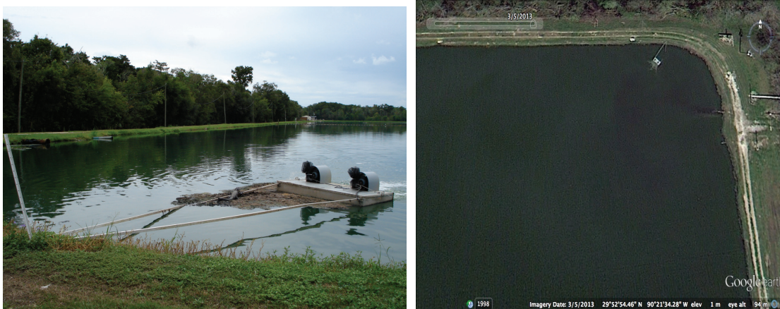
Figures 6 and 7 – (L) The Lagoon Master Aerator that has excavated all the sludge islands at the inlet of the 60 acre wastewater lagoon in southern Louisiana. (R) A satellite view of the same inlet lagoon corner with aerator in place. No islands exist in this photo. (Note: Yes that is an alligator sunning on the left stanchion of the aerator.)
