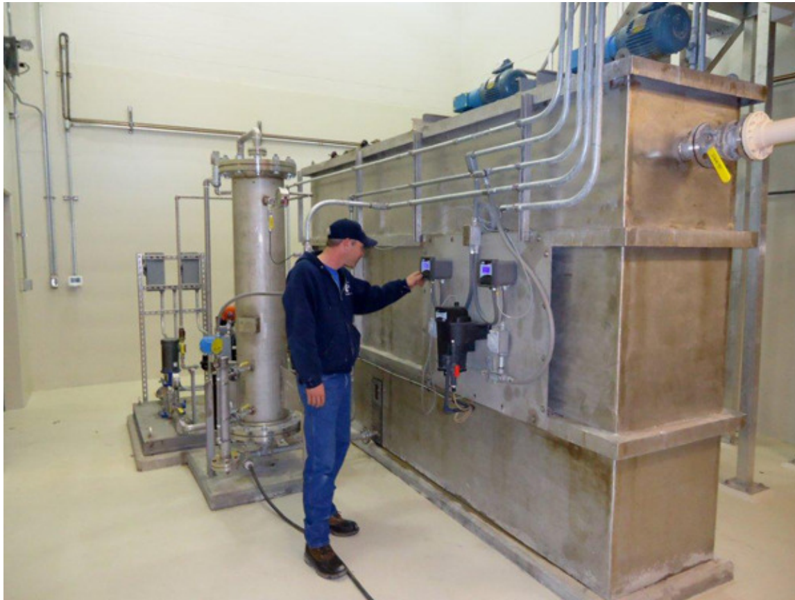
The Clari-DAF system's use of a mechanical skimmer significantly reduces the reliance on former chemical treatment and related higher costs. View of the utility's 'mini Clari-DAF plant' used for training operating personnel.
