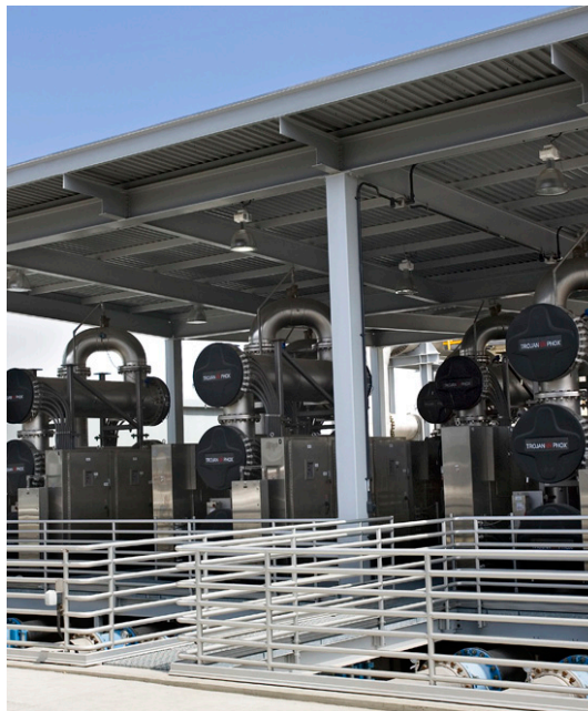
This TrojanUVPhox™ at the Orange County Water District removes NDMA and any other wastewater-derived contaminants that may be present in MF and RO-treated secondary effluent.
