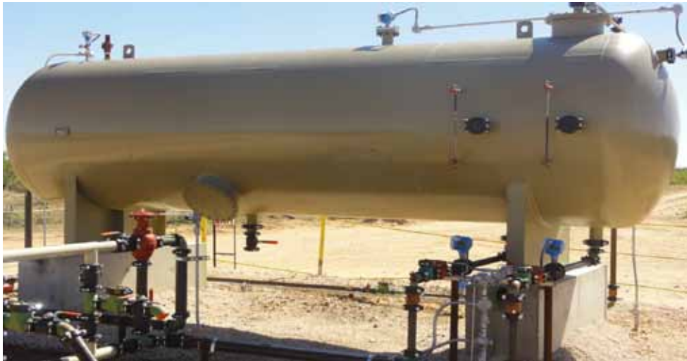
Figure 1: In a separation vessel, oil and water separate, with oil moving to the top and water to the bottom. Capacitance level switches are used to detect the oil/water interface.
