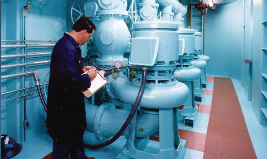
Four Smith & Loveless Flooded Suction Non-Clog Pumps dutifully work, day-in and day-out in this CAPSULAR® Pump Station.
