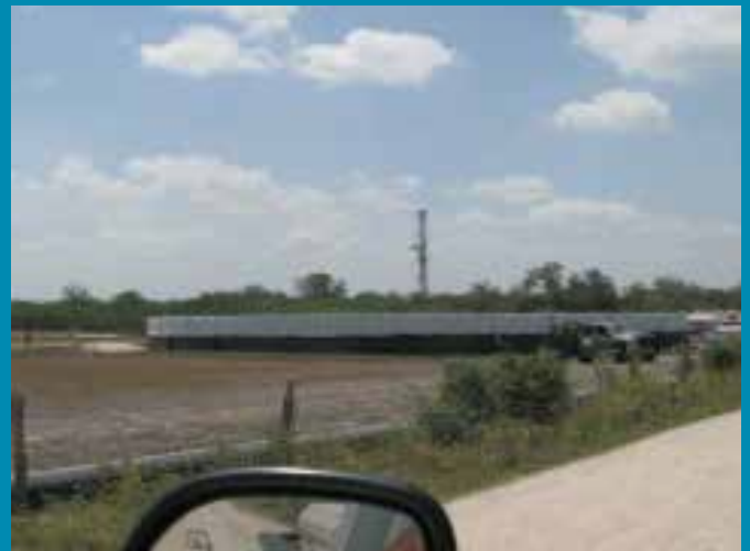
40,000 barrel temporary storage tank
