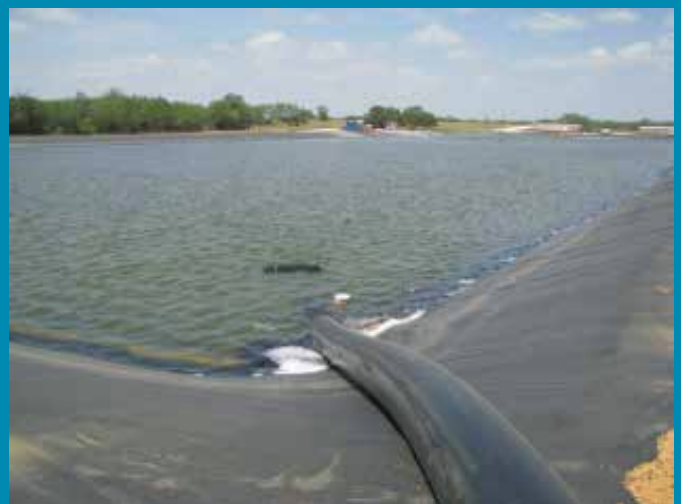
300,000 barrel temporary frack pond
