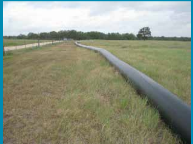
7.5 miles of 18" HDPE piping
