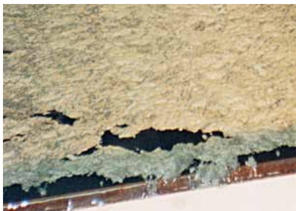
This floating blanket of membrane-fouling sludge is a security blanket for membrane filters.
