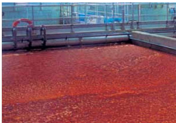
The next step for this sludge produced by a Clari-DAF® system is dewatering where higher cake solids result in lower disposal cost.
