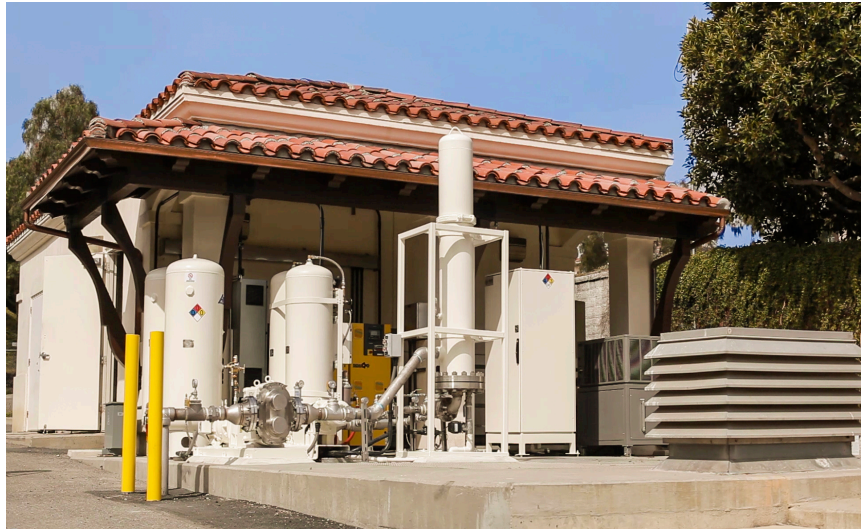
Anue Water Technologies Force5 ozone-based process for H 2 S control at the Talega site.
