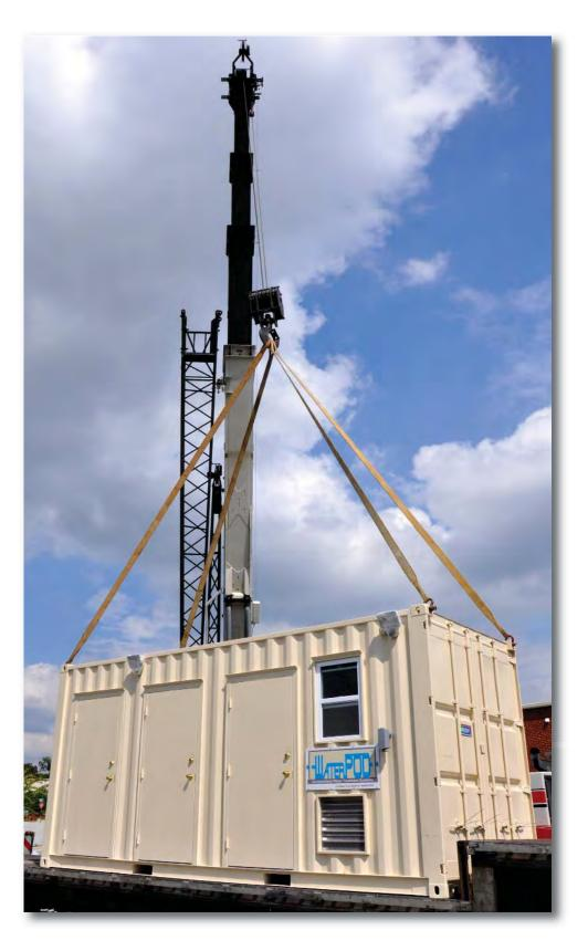
WaterPOD Containerized Treatment Units from AdEdge Water Technologies have been developed to meet the growing U.S. and International demand for small footprint, cost-effective modular water treatment installations. The fully integrated, pre-engineered, pre-wired, packaged water treatment solution combines system performance with economy resulting in an ideal solution for sites where space, cost, and schedule are critical.
