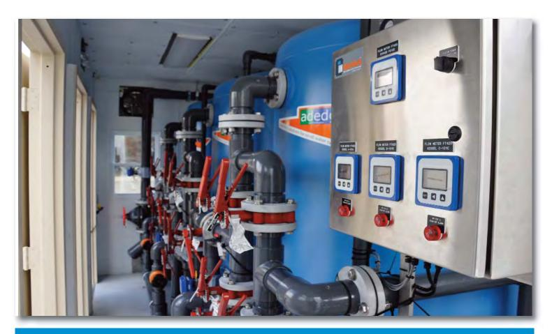
The treatment systems are designed, custom built and delivered inside the pre-manufactured and customized water tight enclosure. The unit is constructed of painted carbon steel with coated steel overlay on the wooden floor and can include multiple other customizable options including insulation, lighting, ventilation, pedestrian doors, windows, HVAC unit to meet site specific and weather requirements.
